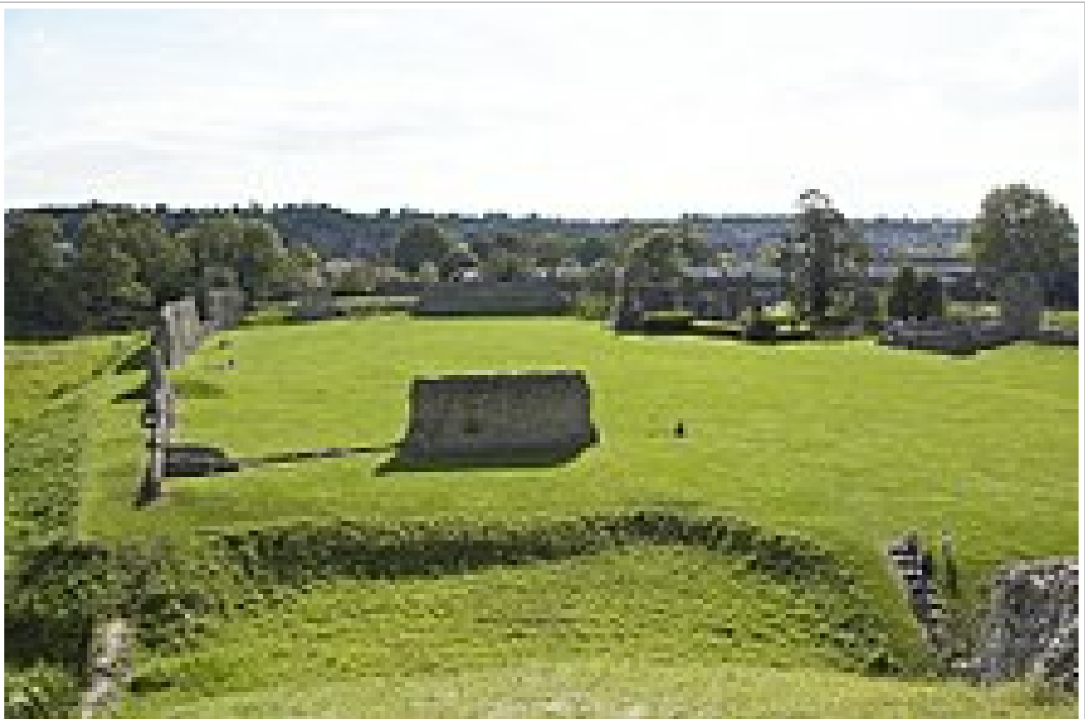
The ruins of Berkhamsted castle (viewed from its Norman motte) and Berkhamsted Common were the location of two successful early preservation events in the nineteenth century. (Enlarged: A train passes Berkhamsted castle, on an embankment that was once part of the castle's outer defences.)
